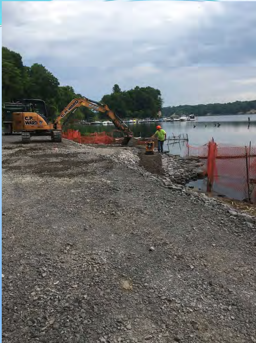
Area B - Stone Dust Trail Construction
