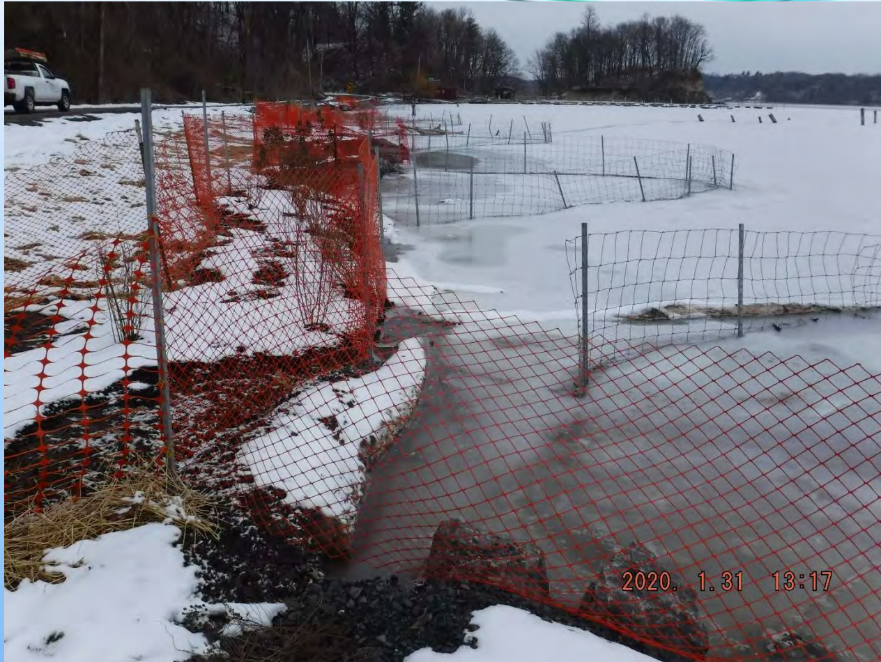
Area B – Rock placed, coir logs placed, goose barrier and carp barrier placed
