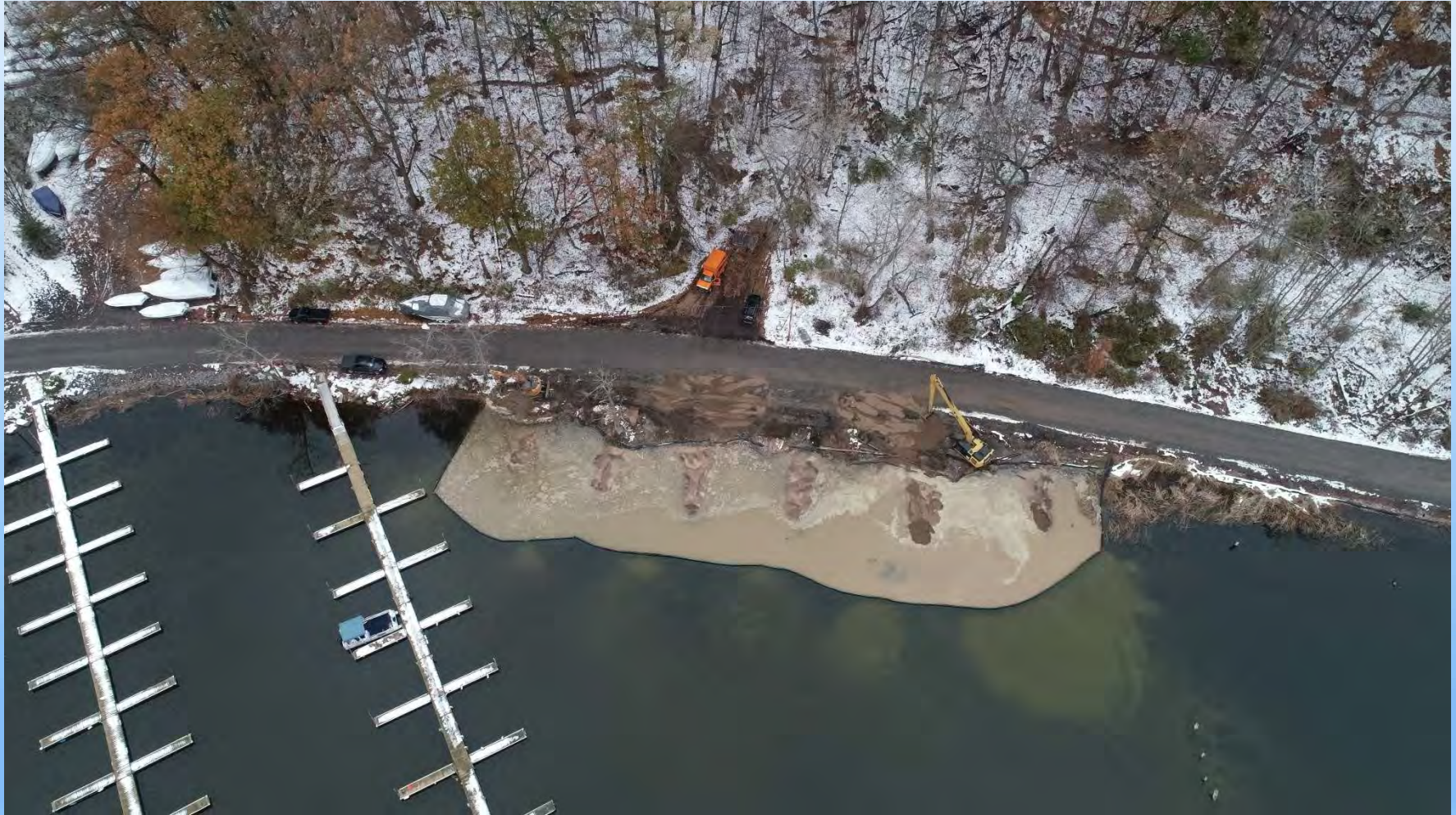
Area B under Construction – Turbidity Curtain in Use
