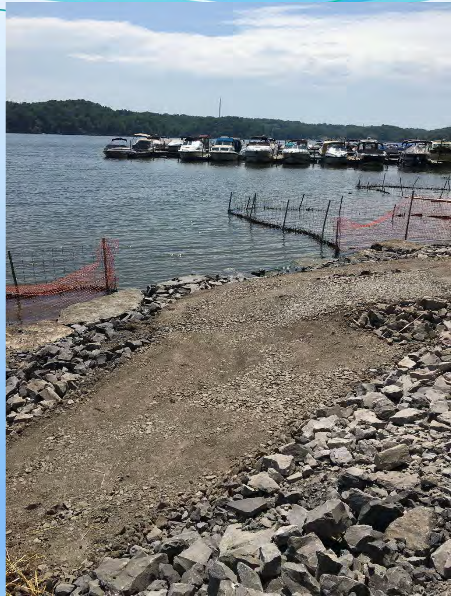
Area B - Stone Dust Trail Construction
