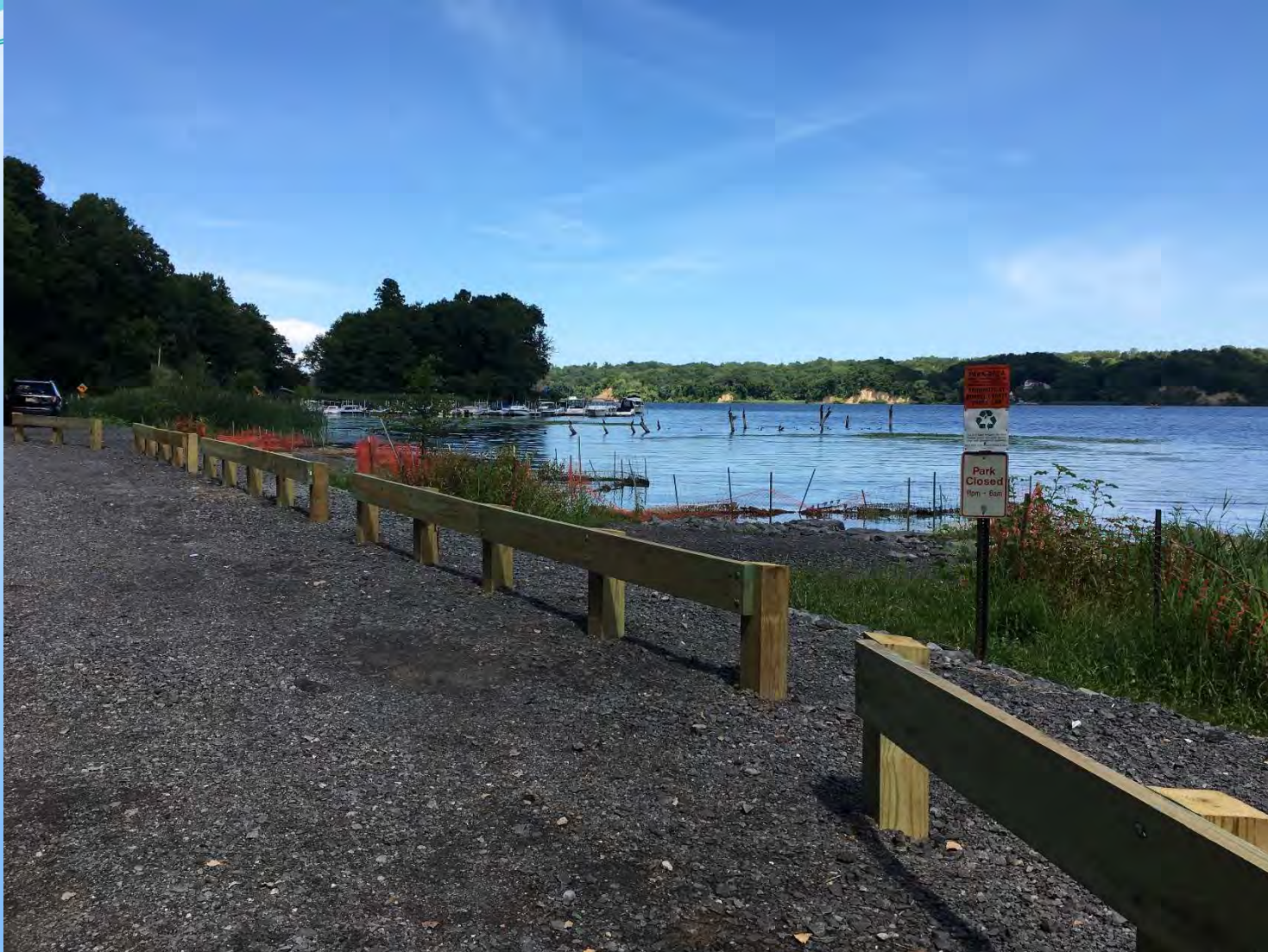
Area B - Timber Parking Guide Rail Installed
