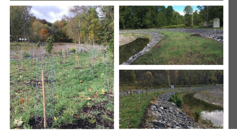
Riparian Benches were installed to slow velocity through bend in stream
