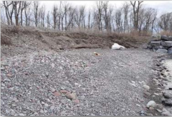
Wayne County shoreline stabilization project. Photo credit: Wayne County SWCD
