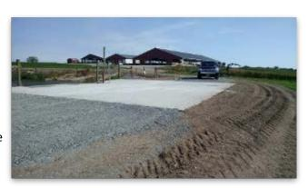
concrete will prevent leaching into the ground and allow for easy cleanup if there is a spill. The pad is sloped towards the lagoon, so that if a spill does occur it will flow back into the lagoon and not off the pad into the surrounding area. The total cost of this project was \$9,365.88 of which FLLOWPA paid \$7,024.41 (75% of total project cost) and the farm paid the remaining balance.
