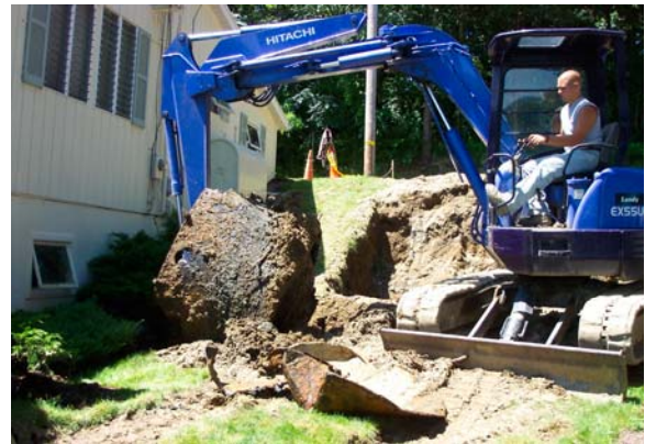
Replacement of failed septic tank in Schuyler County
