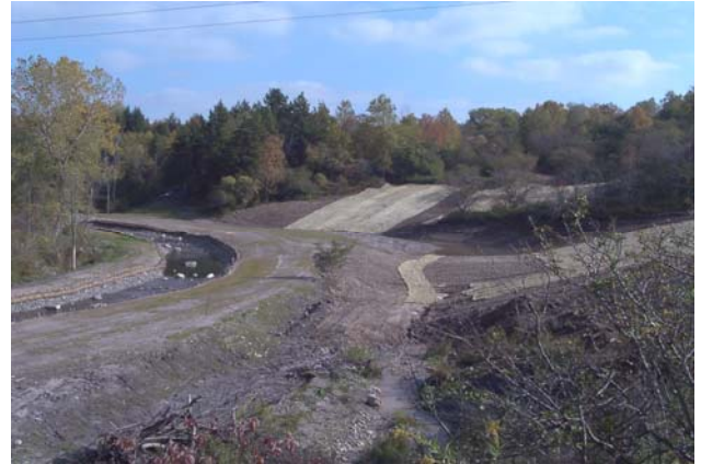
After: Stabilization measures installed
