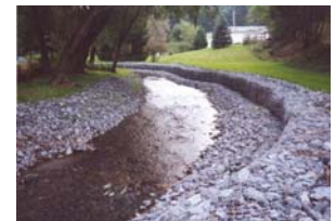
Streambank stabilization in Wayne County
