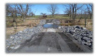
**The George Family Farm** completed a heavy use pad for the calf hutches. Originally, runoff from the hutch area was not controlled and drained to the farm access road where it mixed with roof runoff. The farmstead is only 2000 feet from Cayuga Lake. The hutch area were moved to an improved site and vegetated treatment area was installed downslope to treat runoff.
